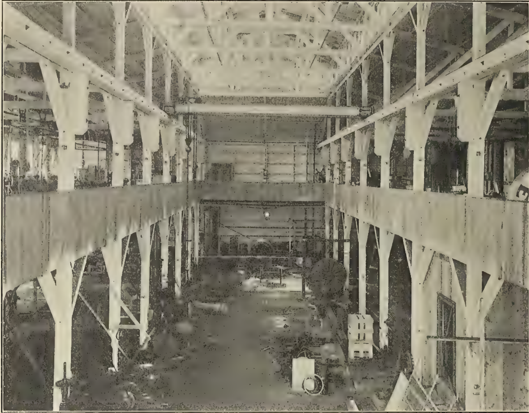
INTERIOR OF THE JERSEY CITY SHOP OF THE GRISCOM-SPENCER COMPANY.
